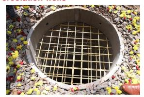
Percolation wells are designed to capture rainwater so that the groundwater table is restored, conserved and recharged as the created percolation and filtration environment triggers natural aquifers.
